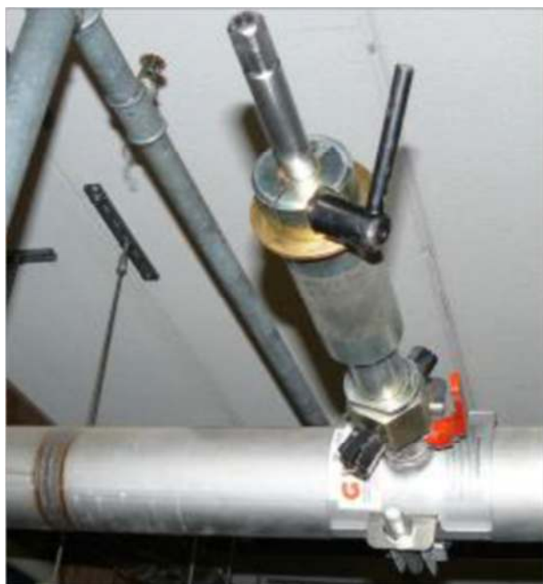
Picture 3: Placing the drill
