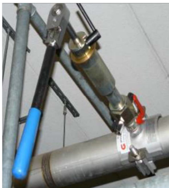
Picture 4: Ready for drilling
