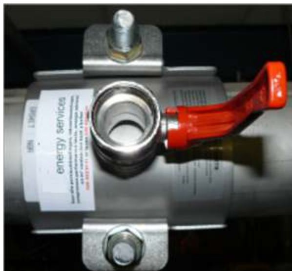
Picture 2: Mounting of a clamp
